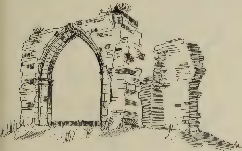
FIG. 1454.—Dron Church. View from South-West.
